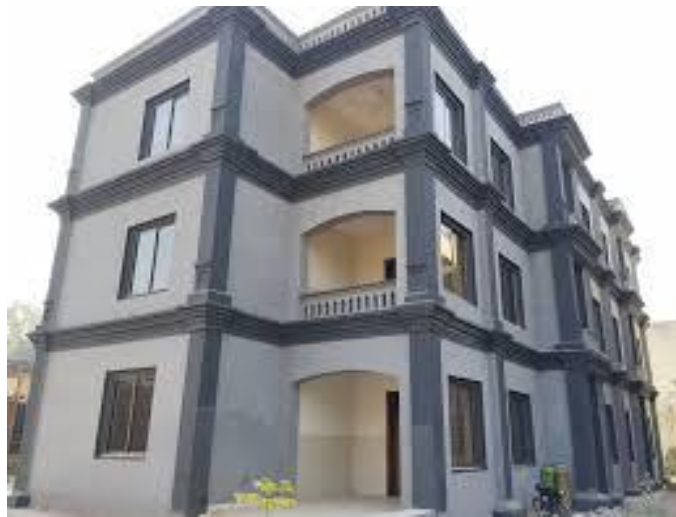
Construction of new hostel
