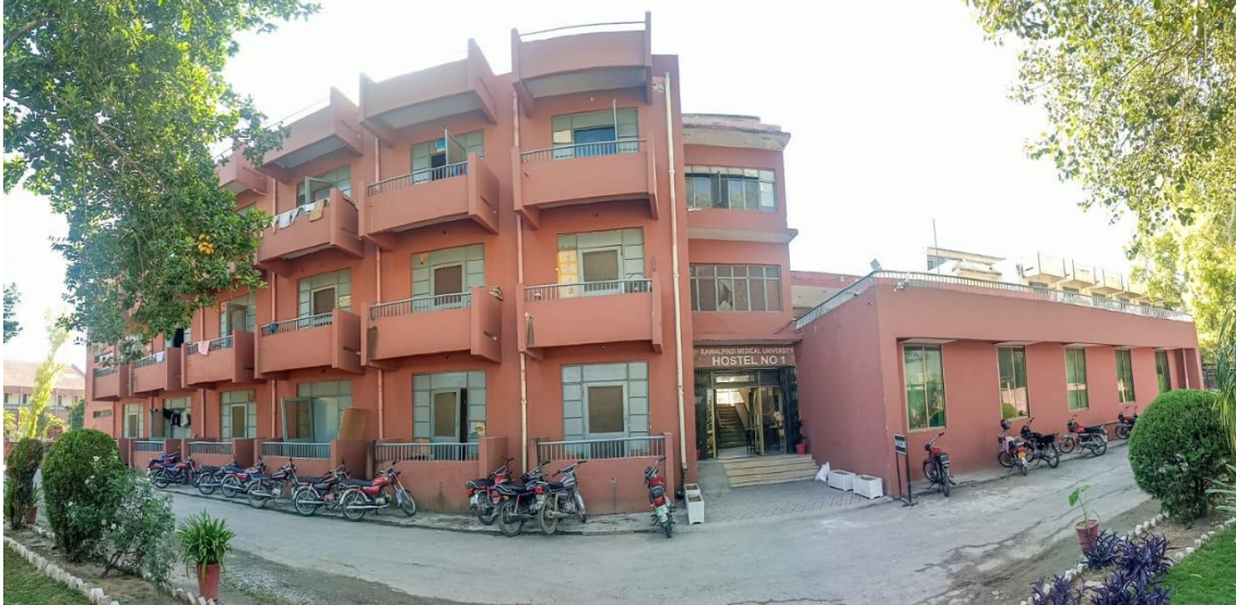
Renovation of Existing Boys Hostel
