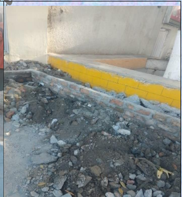
Construction of patient Benches using the debris generated during construction work.
