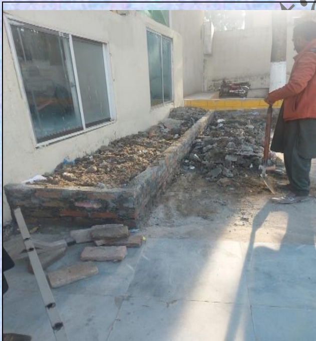
Construction of patient Benches using the debris generated during construction work.
