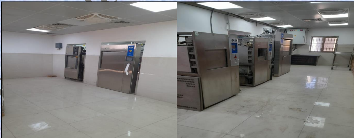
Theatre Sterile Supply Unit has been installed in Modular Operation Theatre for efficient and effective sterilization of Instruments and linen.
